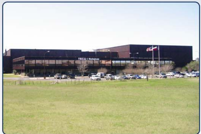
The TECO-Westinghouse Motor Company manufacturing and global R&D facility in Round Rock, Texas.
