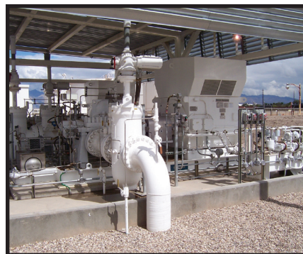
These seven 2500 HP induction motors driving pipeline pumps provide additional refined product capacity to the southwestern part of the United States.
