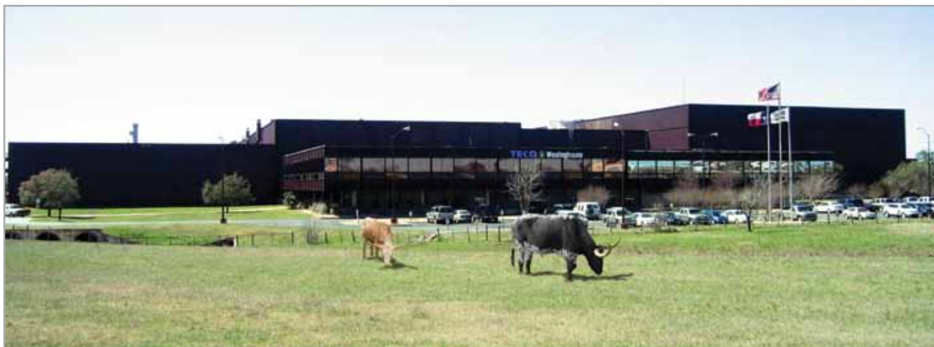
TECO-Westingshouse North American Headquarters in Round Rock, Texas, USA
